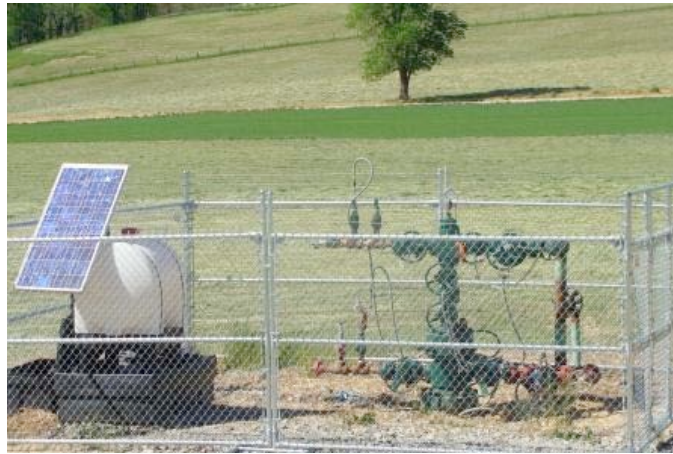
Figure 11: Completed Wellhead Site
