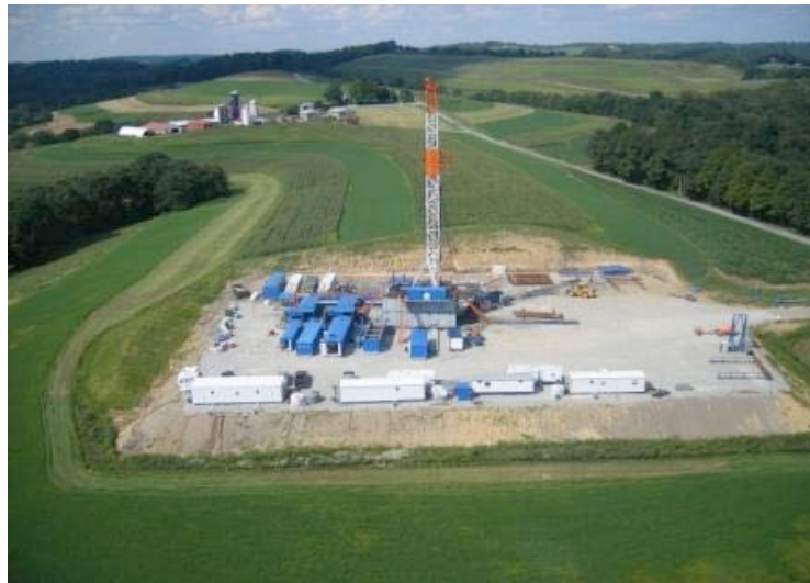
Figure 9: Well Site during Drilling
